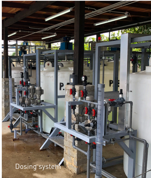
DAF system using DIACHLOR coagulant
